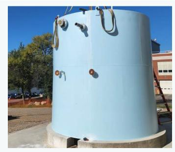
Pre-treatment tank (clarifier) for pilot testing
